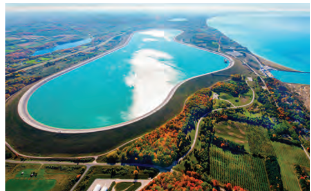
Ludington Pumped Storage Plant. Photo credit: Consumers Energy
