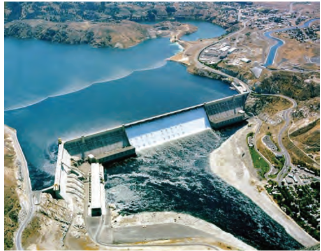
Grand Coulee Dam. Photo credit: U.S. Bureau of Reclamation
