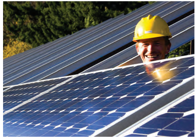
Installing solar panels. Photo credit: Oregon Department of Transportation
