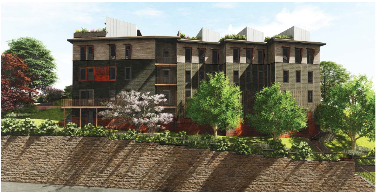
Fort House is a five-unit residence in the Highland Park Neighborhood of Roxbury, MA. The design/builder, Placetaylor, expects to complete the project in Fall of 2019 with a predicted site EUI of 13 kBtu/sf/yr. The project will achieve Zero Energy for less cost per square foot than this report's baseline small residential building. Image credit: Placetaylor.
