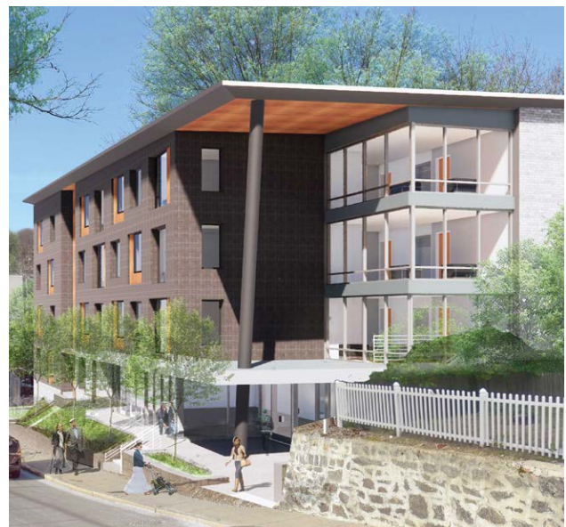
E+ 273 Highland St, Boston - Multifamily Residential (23 units) LEED Platinum and net energy positive (HERS 37 / with solar PV, -3). Rees-Larkin Development with Studio G Architects. The E+ Green Building Program is an initiative of the Department of Neighborhood Development and the BPDA. Image credit: Studio G Architects.
