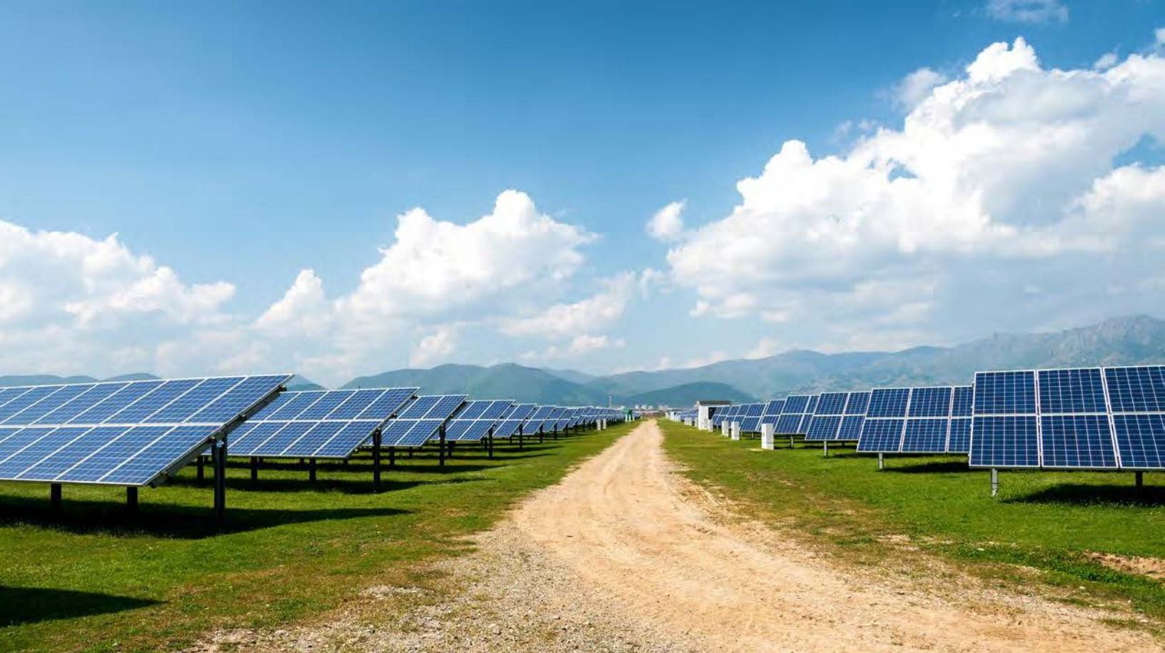
Panoramic view of solar panels.
