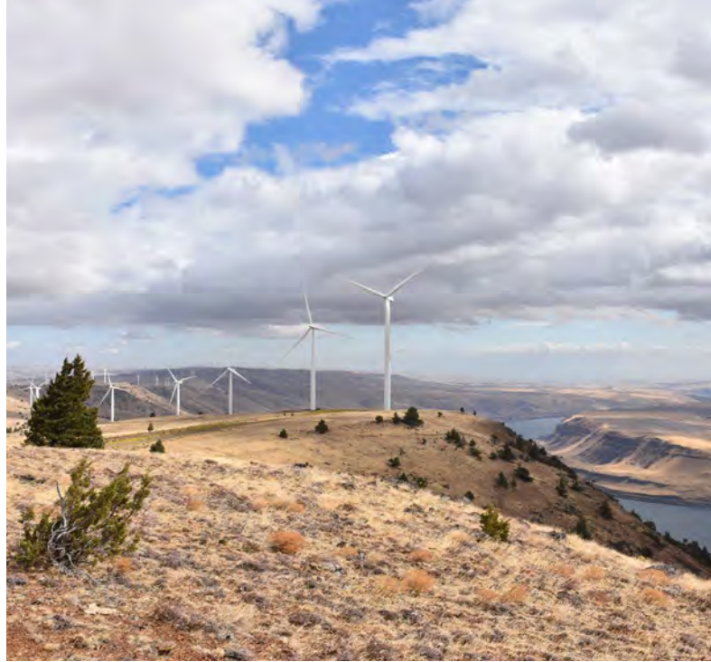
Wind turbines, Goldendale, WA. Clean Energy Transition Institute
