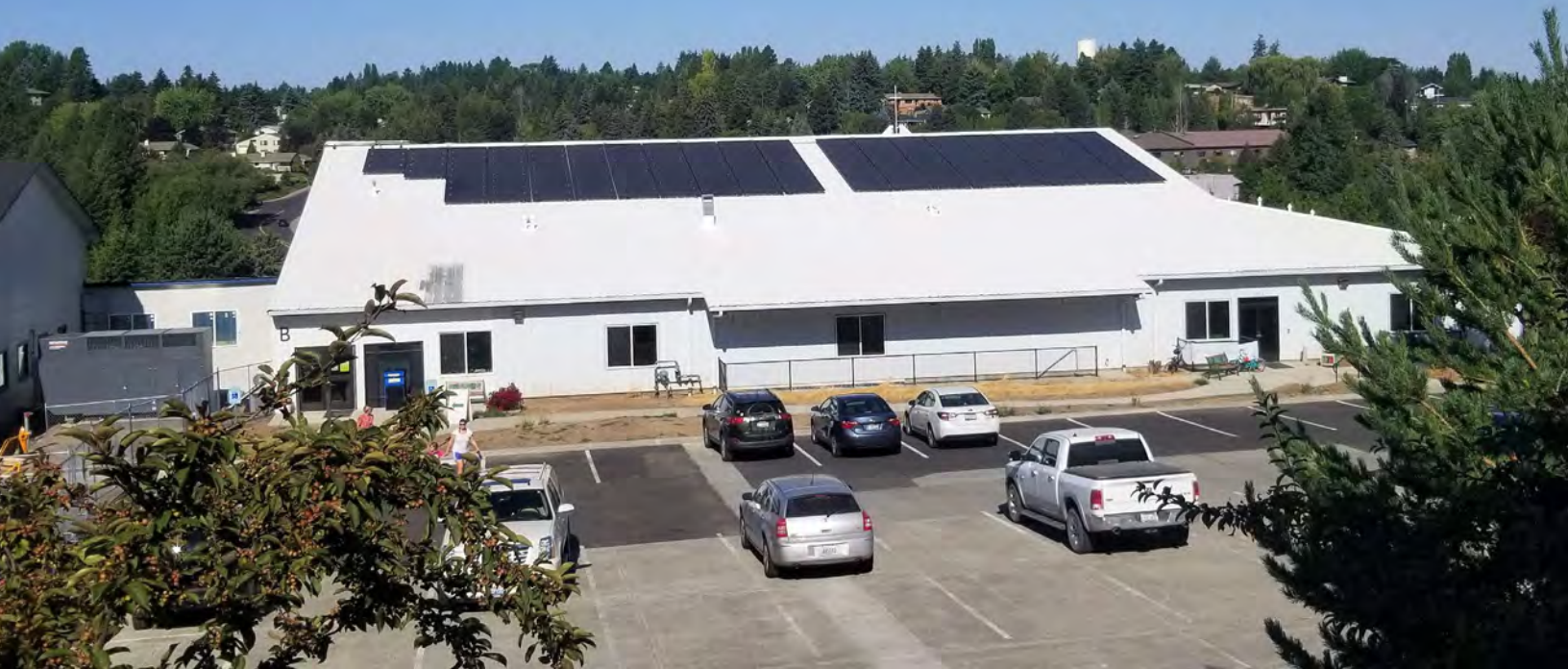
Solar power system on the new Parks, Recreation and Senior Center building in Pullman, Washington. Funded in part by a grant from Commerce's Energy Efficiency and Solar Grant program. Department of Commerce
