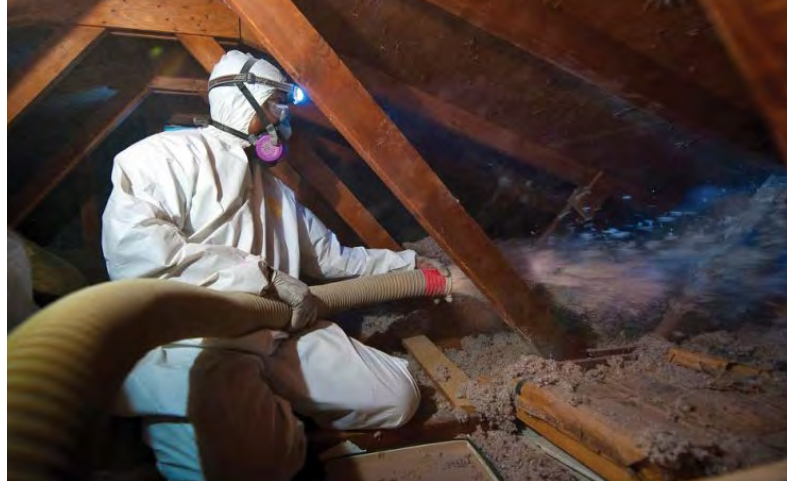
Attic insulation with Weather Assistance Program. Department of Commerce
