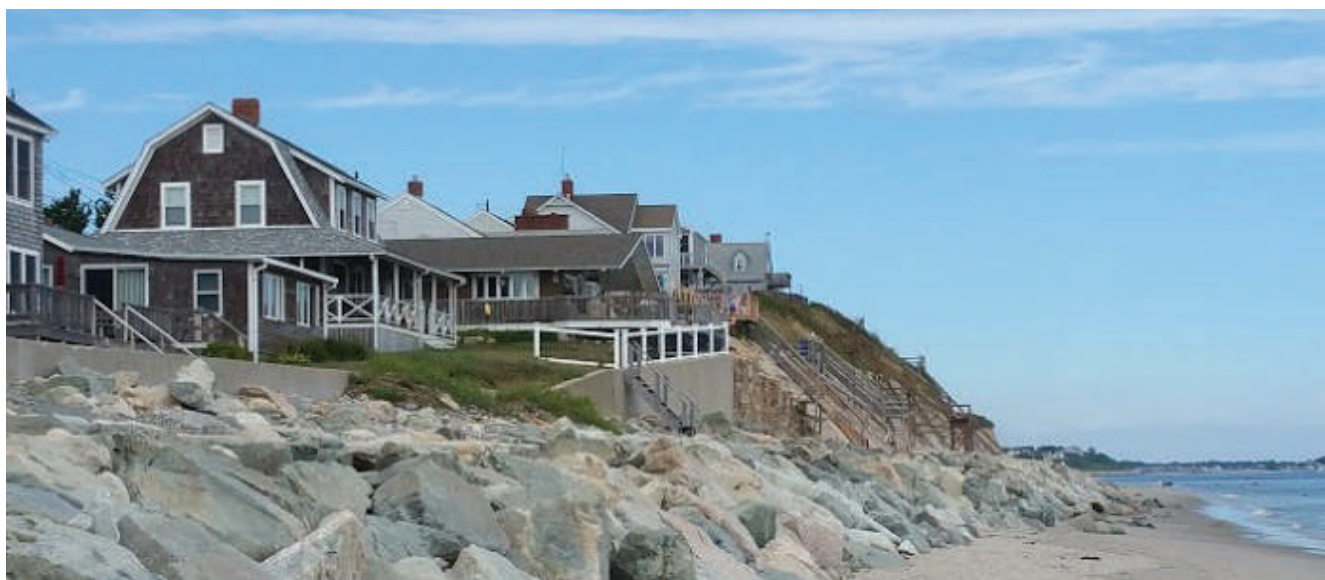
Photo courtesy of Carri Hulet, CBI.
