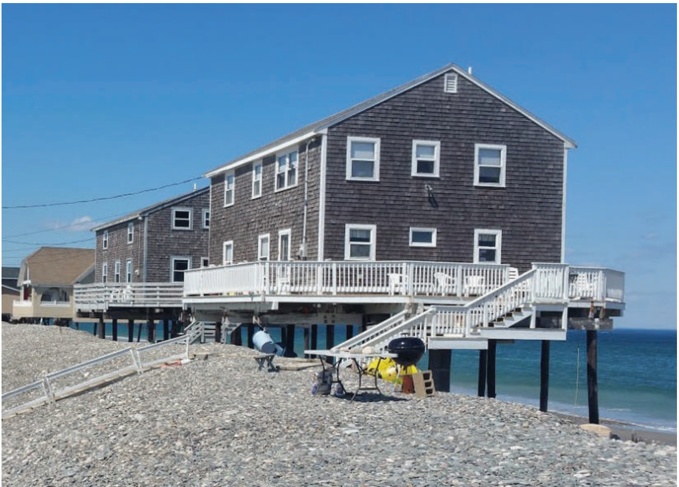
Photo courtesy of Carri Hulet, CBI.
