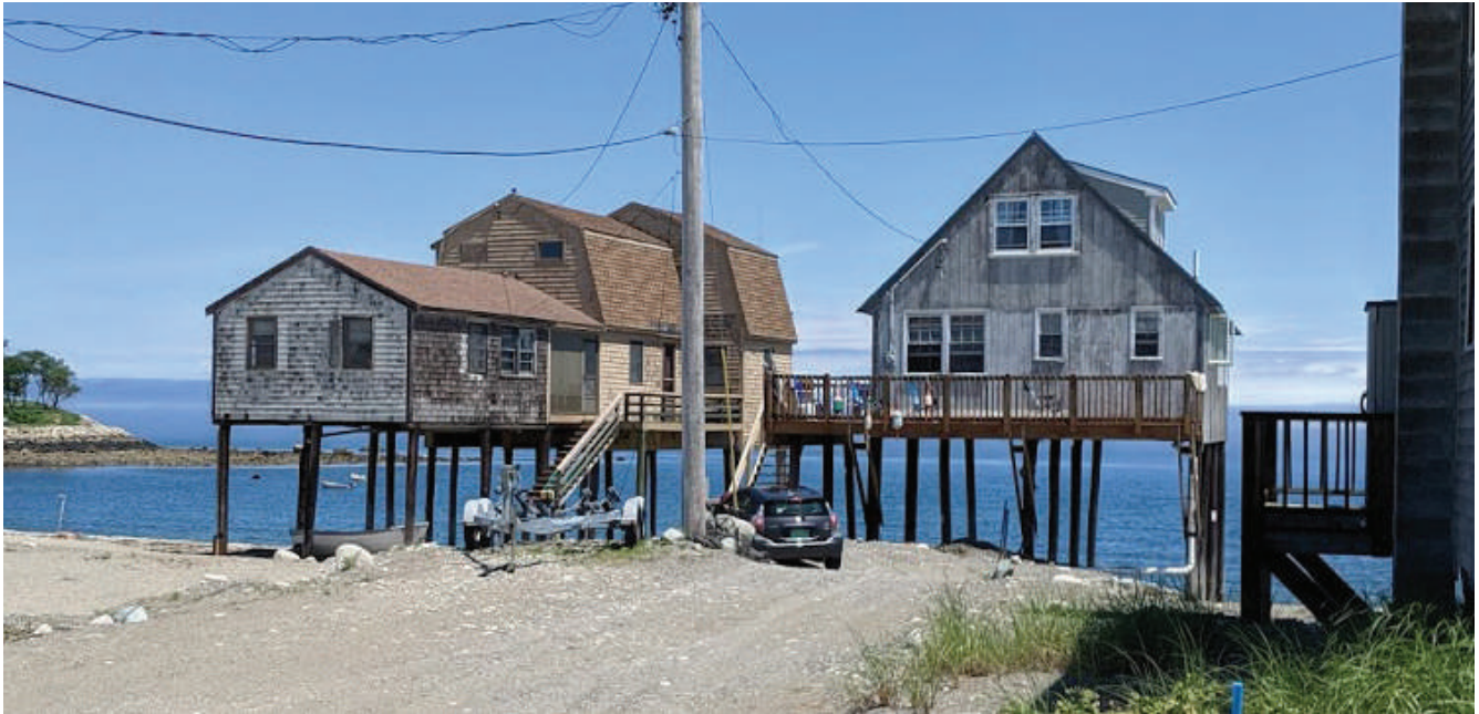
Photo courtesy of Carri Hulet, CBI.
