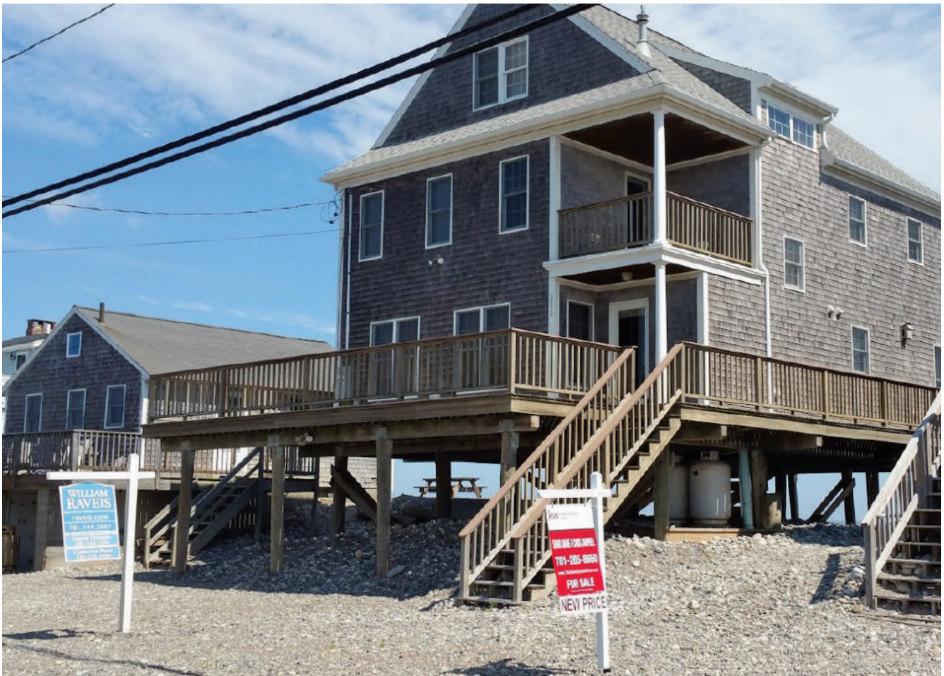
Photo courtesy of Carri Hulet, CBI.
