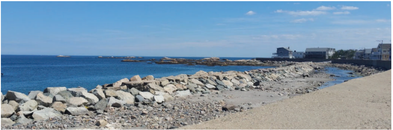
Photo courtesy of Carri Hulet, CBI.
